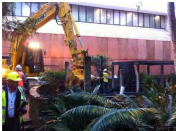
Construction work well and truly advanced at the Sydney Gateway Facility
